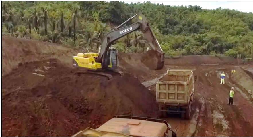
Figure 6-6. Loading of removed topsoil.
