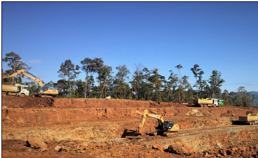
Figure 6-7. Loading of ore to 18-ton capacity dump trucks.
