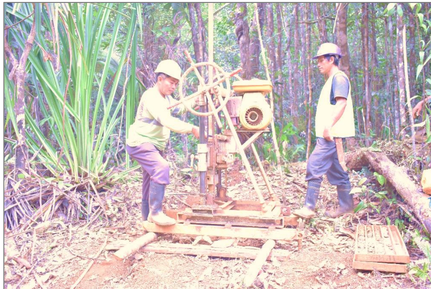
Figure 10-6. MMDC in-house drilling.
